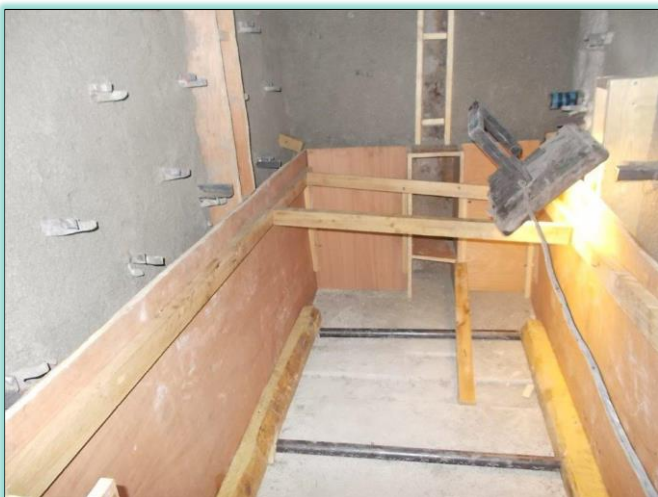
Lower shuttering in place and supported
