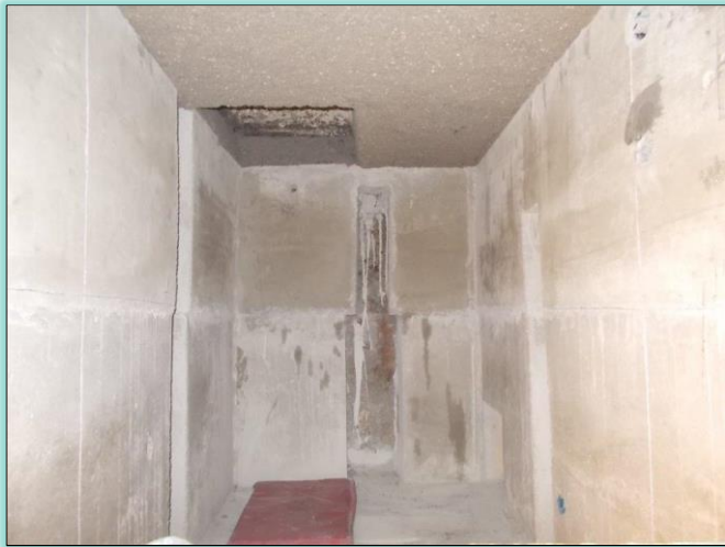
All walls casted and roof rammed in plastic (mouldable) refractory
