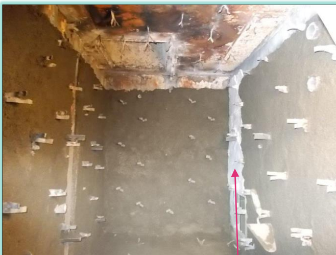
Insulating layer rammed up. Note the inner layer of ceramic wool
