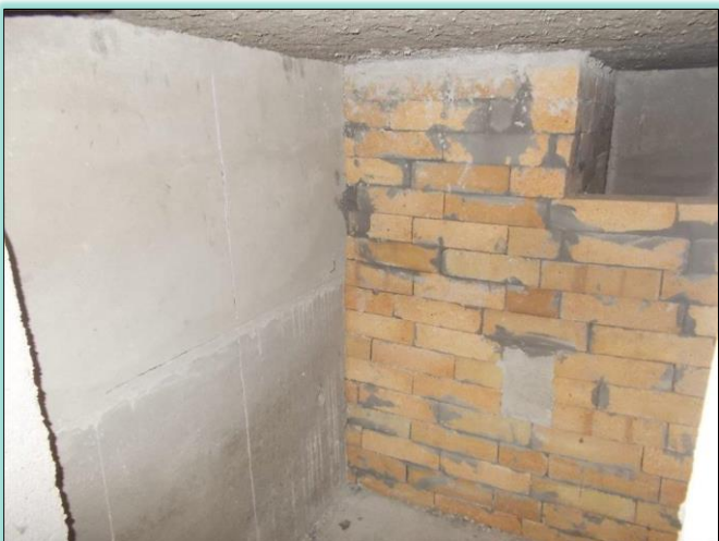
Refurbishment completed. First chamber with view into second chamber
