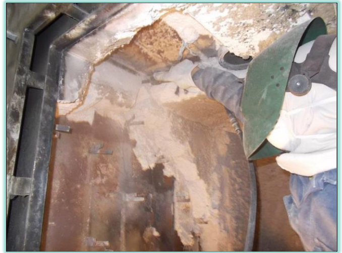
Removing all refractory and lining
