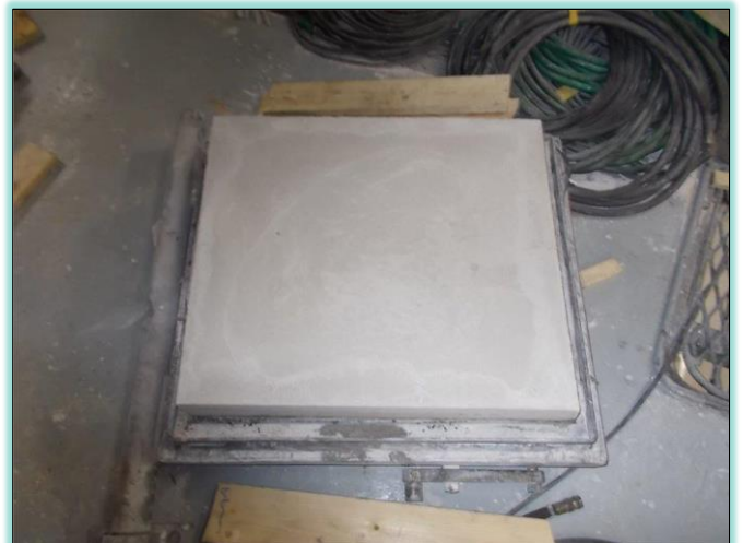
Door after refurbishment
