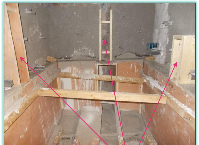
Casting of lower part Note the slots to support wall bricks
