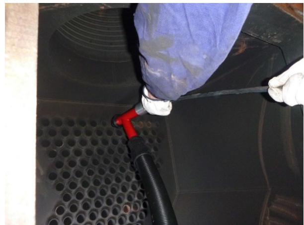
Figure 7 Cleaning of horizontal boiler
