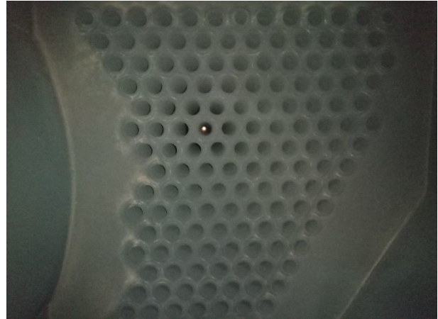
Figure 3 Horizontal boiler prior to cleaning
