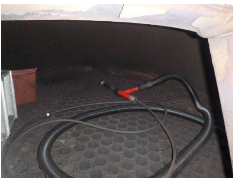
Figure 5 Cleaning of vertical fire tubes where access only is allowed from above
